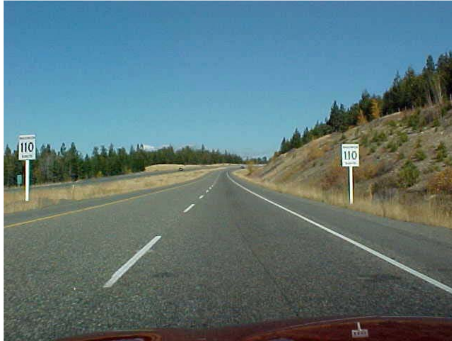
Figure 3. Operating speeds indicate the 110 km/h limit on this rural freeway should be raised to 120 km/h.
