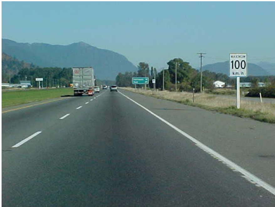
Figure 4. Operating speeds indicate the 100 km/h limit on this rural freeway should be raised to 110 km/h.
